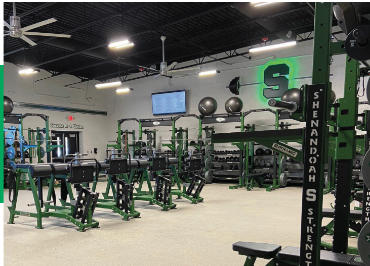
Design Build construction of new Weight Room
