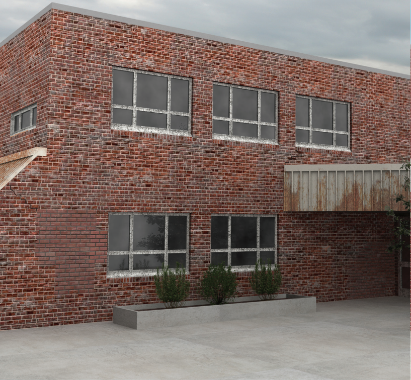
Before FAÇADE RESTORATION
