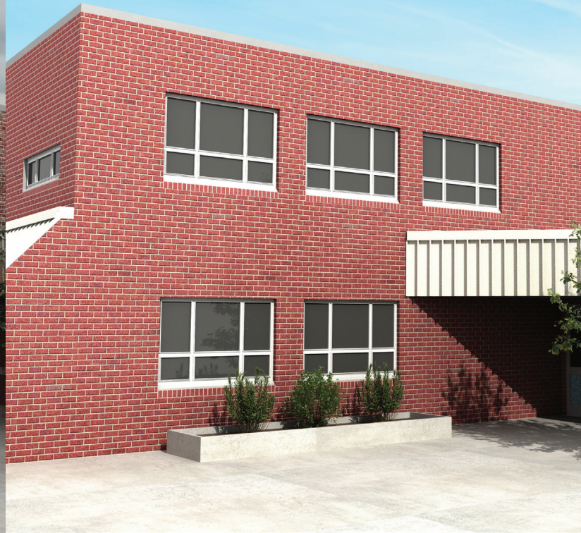
After FAÇADE RESTORATION
