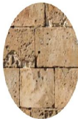
SPALLING AND EROSION
