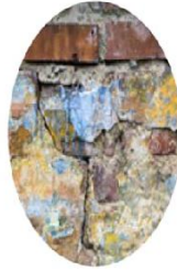
EFFLORESCENCE
