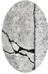
CRACKS – HAIRLINE OR LARGER
