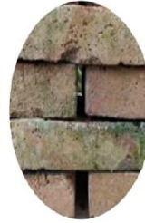
LOOSE OR MISSING MORTAR
