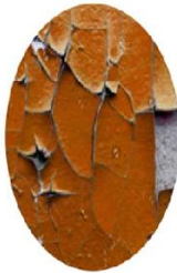
FLAKING OR PEELING PAINT
